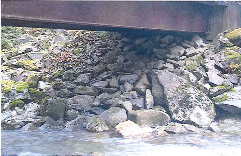
CK2260 Right Abutment
