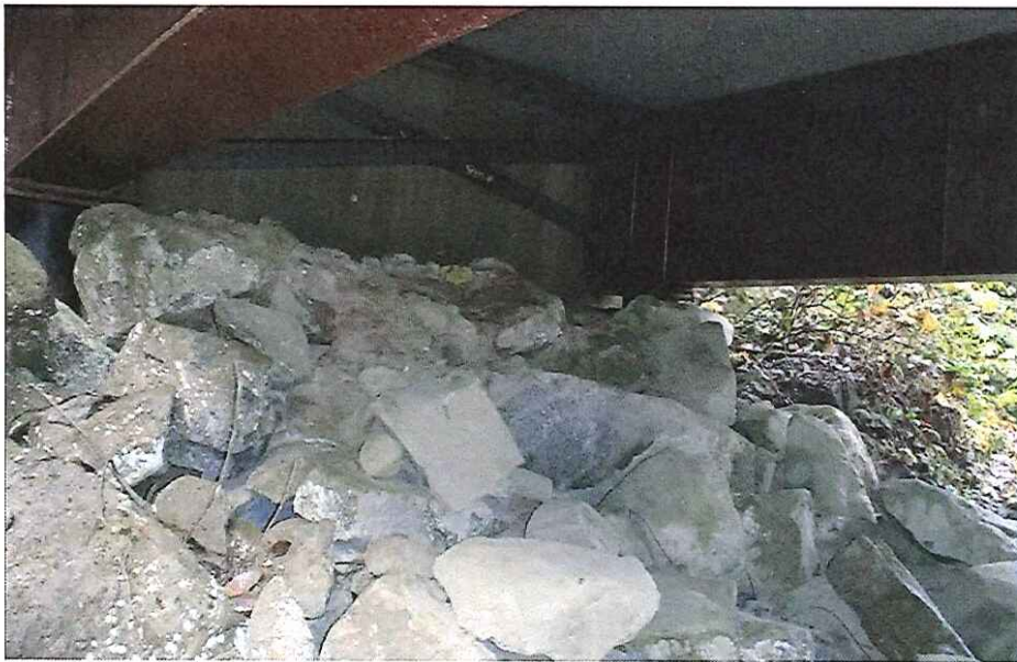
CK2260 Left Abutment
