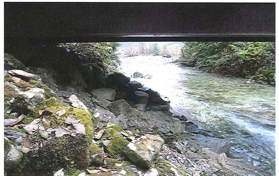
CK2260 Left Abutment Rip rap
